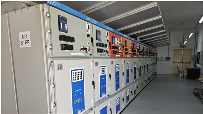
The 11kV switchgear in the TRP substation.
